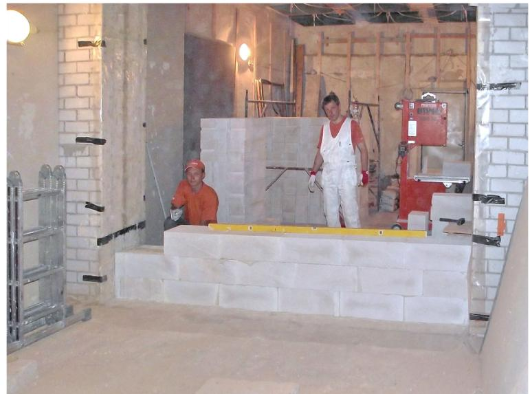
Fig.1. Built in of the sample No. 506-1 in the building acoustics chamber's test opening.
